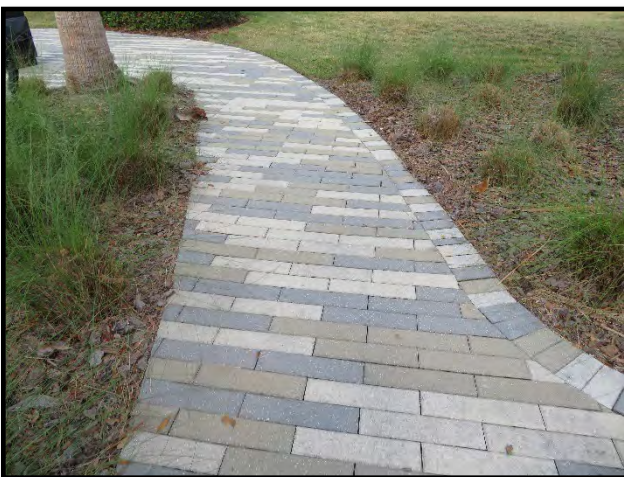
Masonry paver pool deck
