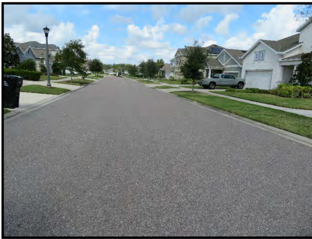
Asphalt pavement at Renaissance Avenue
