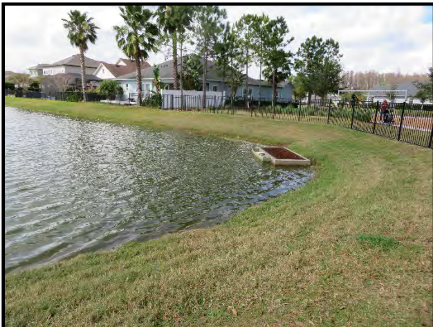
Pond shoreline and outlet structure
