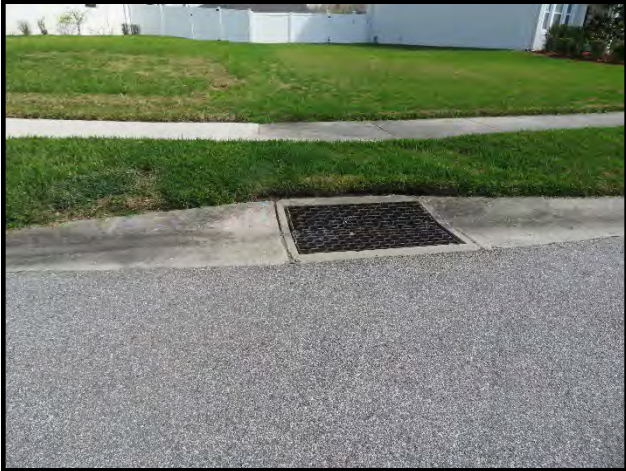
Typical catch basin
