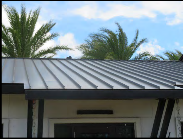
Clubhouse metal roof
