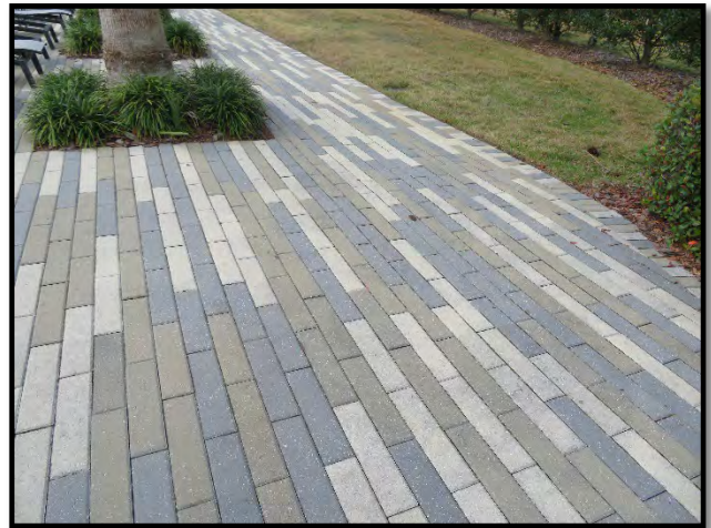
Masonry paver pool deck
