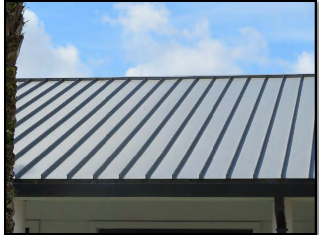
Clubhouse metal roof
