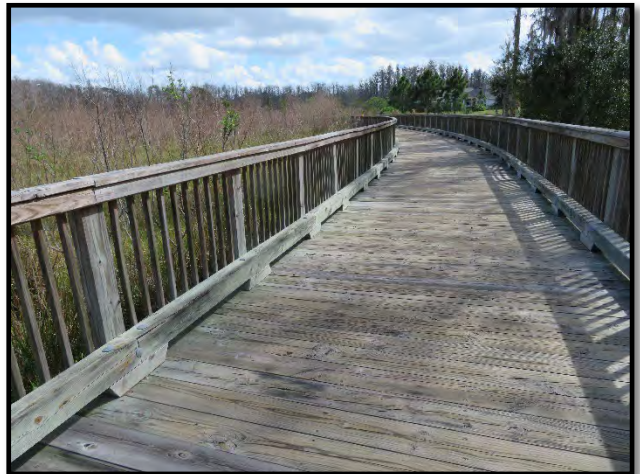
Boardwalk deck and railings
