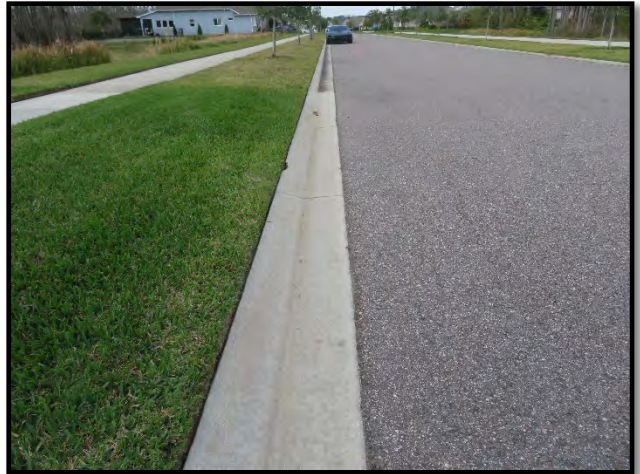
Concrete gutter overview
