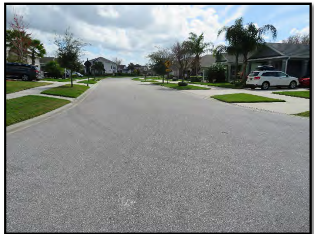
Asphalt pavement at Trails Edge Boulevard
