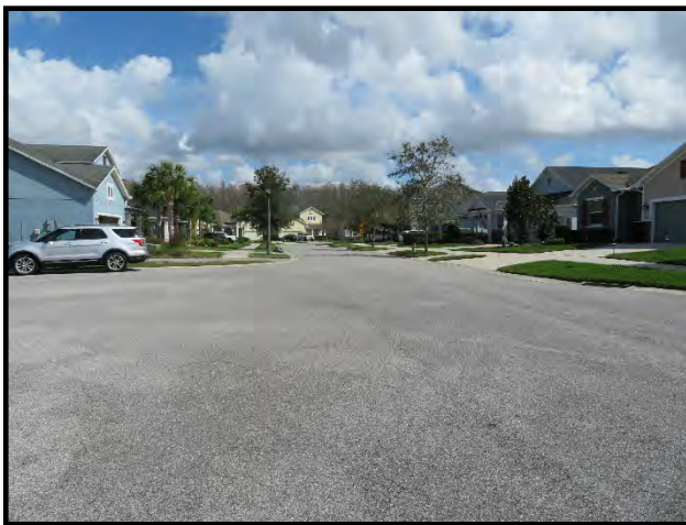
Asphalt pavement at Verona Lane
