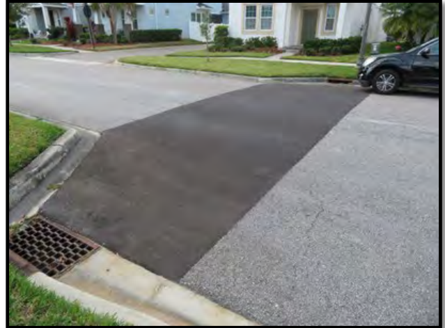
Pavement repair due to subsurface pipe repair at Claymore Street
