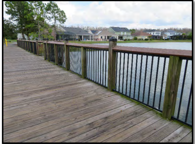
Boardwalk deck and railings
