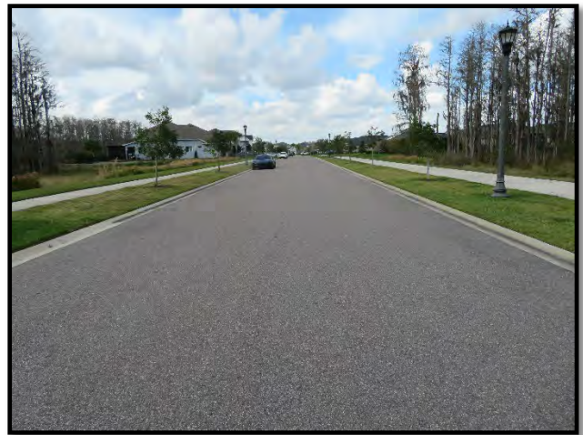
Asphalt pavement at Aviles Parkway
