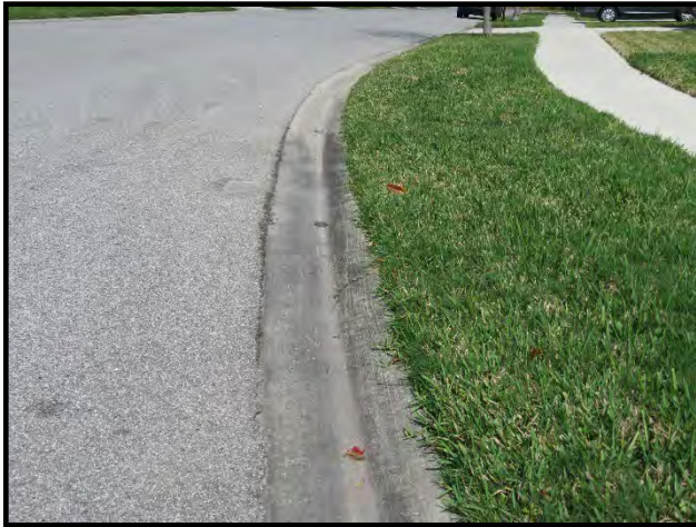
Concrete gutter overview
